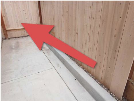
Homeowner's Solution to Major Landscape Drainage Problem was to Hardscape the Area and Install a Curb.
