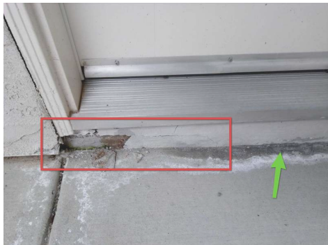
Red Rectangle shows spalling occurring of parge coat & exposing damp sill plate. Green arrow shows moisture damage from pooling water.
