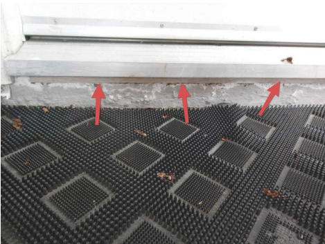
Exposed wood sill plate and messy repair.
